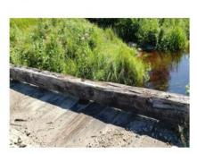
Photo 4: Splits, checks and rot on NW timber curb
