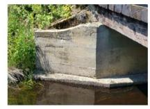
Photo 6: Moderate scaling noted on NW wingwall
