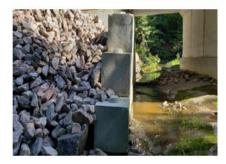
Photo 4: SW retaining wall is leaning towards stream
